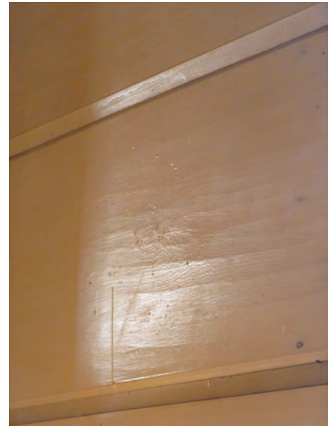
Fig. 12. 1773 hand planed feather edge wall paneling
