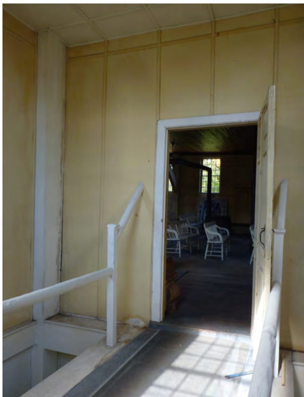
Fig 8. Sloped top rail at upper stair porch entrance to upper meeting hall. A set of 3 riser stairs (Removed 1845) connected the porch to the gallery before the pews were removed and the gallery floor filled in.
