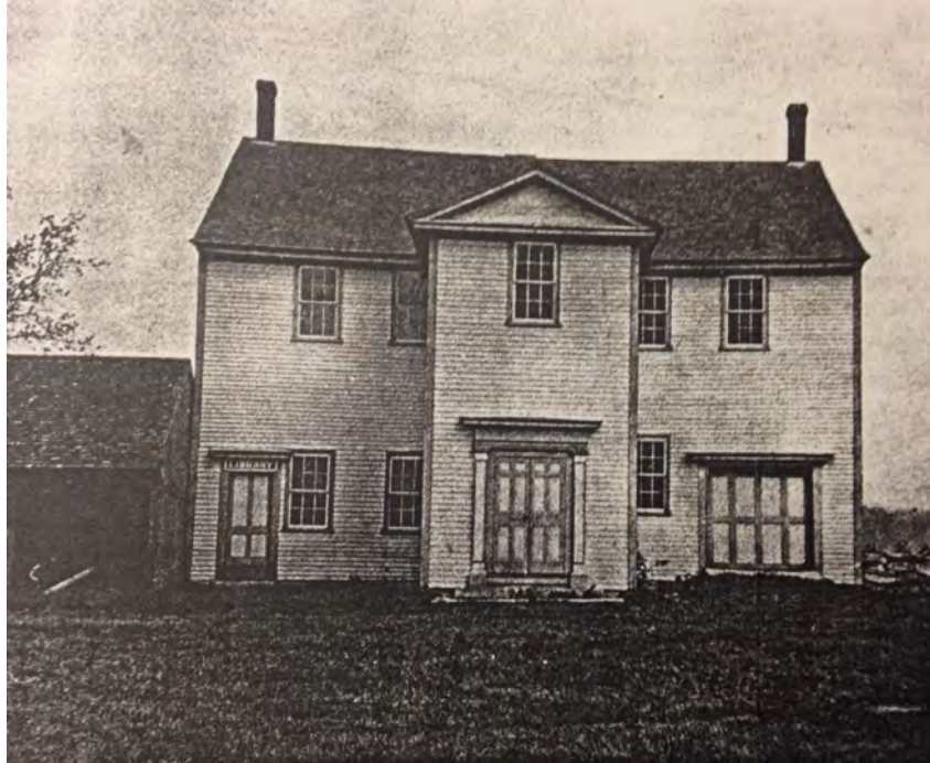
Fig. 2: c. 1897 Town Hall Photo. Horse Shed to the Left
